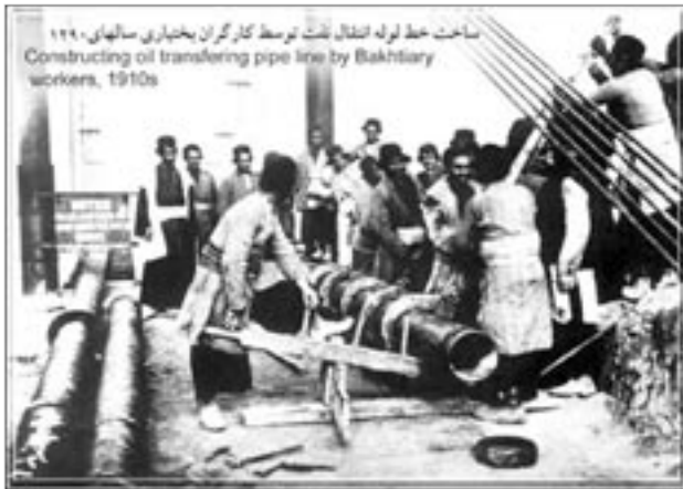
Constructing oil transferring pipe by Bakhtiary workers, 1910s.
