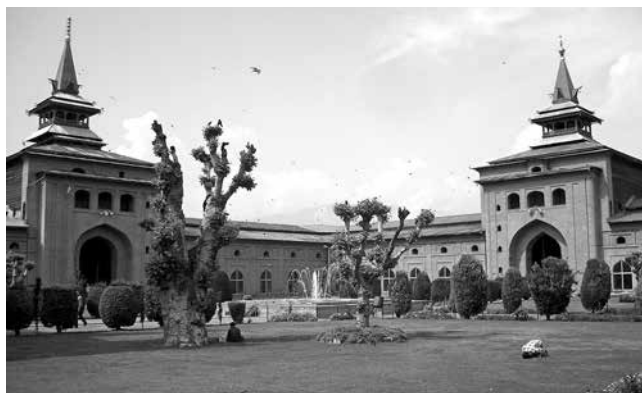
The Grand Mosque of Kashmir (known locally as “Jamia Masjid”) of the city of Srinagar, bears strong Persian architectural influences
